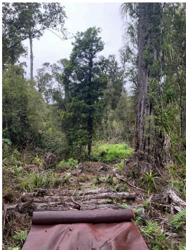
Matting laid prior to spreading of gravel
