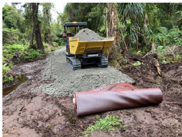
Track Truck used to cart gravel in to track
