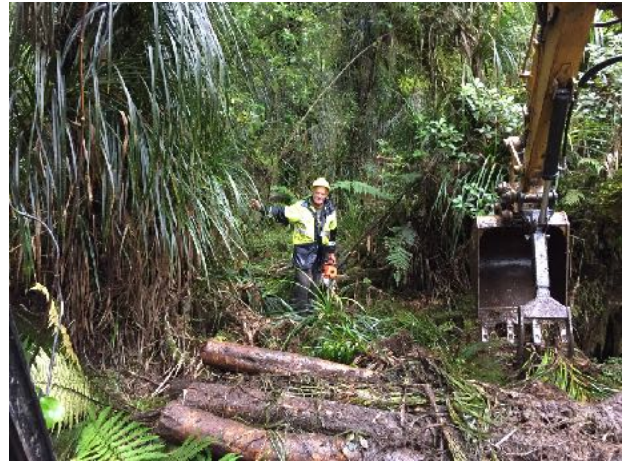
Chainsaw operator clearing ahead of the digger
