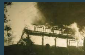
1968 destroyed by fire
